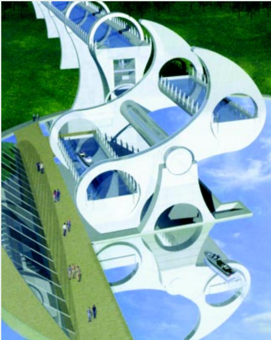
The Falkirk Wheel is a new giant rotating boat lift. It measures 35m in diameter, with an axle length of 28m, and will transfer boats between the two canals, over a vertical gap equivalent to the height of eight London buses.
